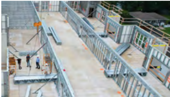
Pre-assembled/pre-fabricated trusses and joists minimize weight and engineering and speed completion
