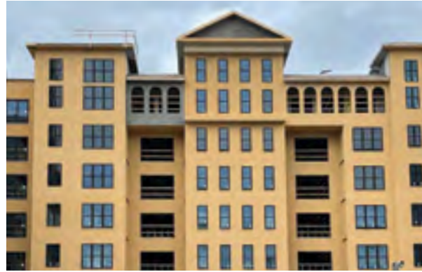
Exterior Finished Wall Panels
